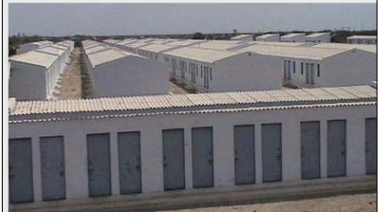
Construction of Worker's Colony for 5,000 workers completed
