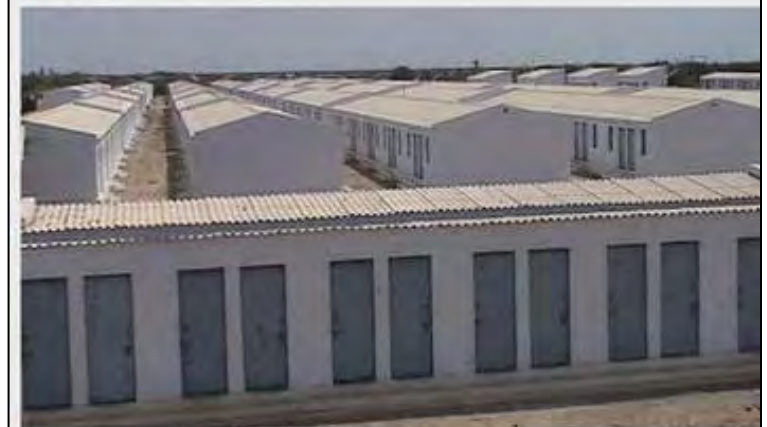
Construction of Worker's Colony for 5,000 workers completed
