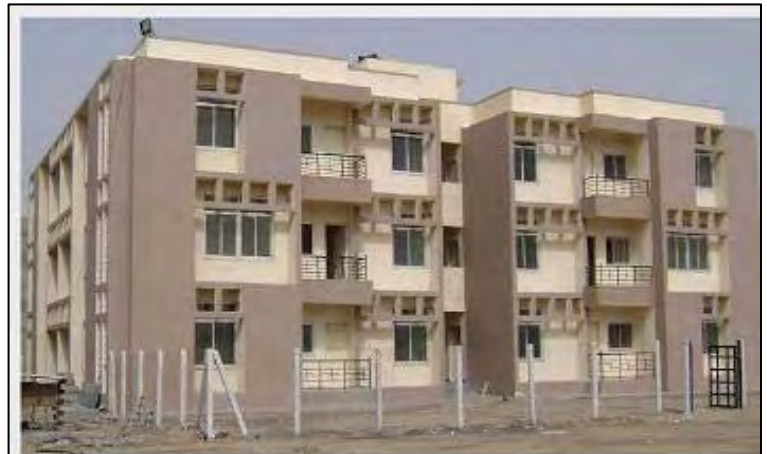
Construction of residential units to accommodate 12,000 families at advanced stage
